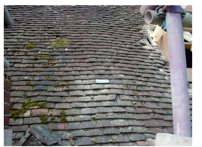
12) Bat-slate in the middle of a plain tile roof. From the ground it's almost invisible.
