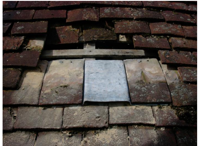
10) Tiles are refitted around the Bat-slate.
