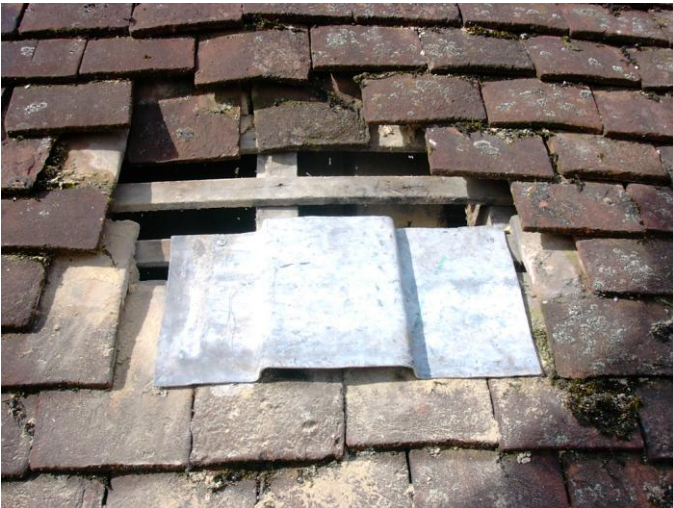
9) The Bat-slate shown here is fitted so that a whole tile will fit alongside it. Where this isn't possible, tiles will require cutting. The Bat-slate is nailed (x2) to the batten.
