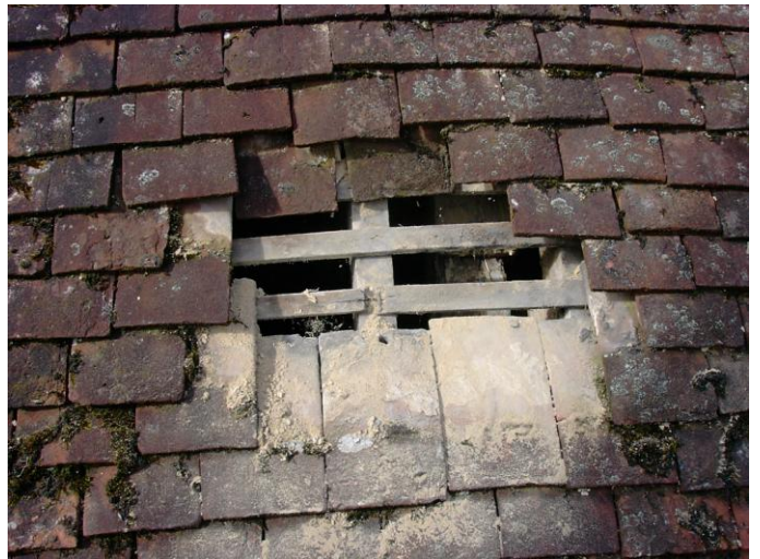
8) A typical place where a Bat-slate might be fitted in an old roof without felt. The Bat-slate will be fitted alongside a rafter, allowing bats to land and crawl out. On a new or re-furbished roof a hole will need to be cut in the felt.
