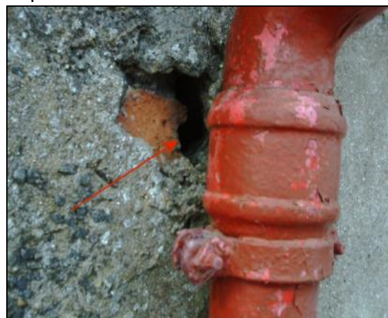
Figure 10: Roost in a hole in a brick wall behind render. © Austin Hopkirk.
