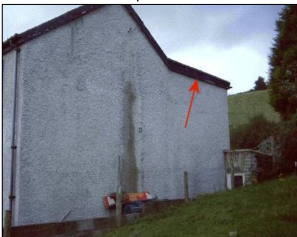
Figure 9: Roost under a soffit just outside Tollymore Park. © Austin Hopkirk.
