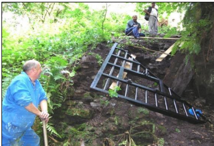
Figure 6: Lower entrance grille being installed.
