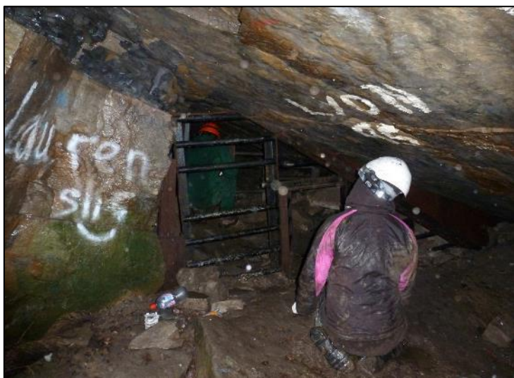
Figure 7: Lower entrance grille after being vandalised.
