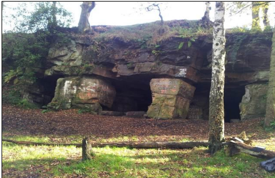
Figure 3: Pillar and stall mining method.
