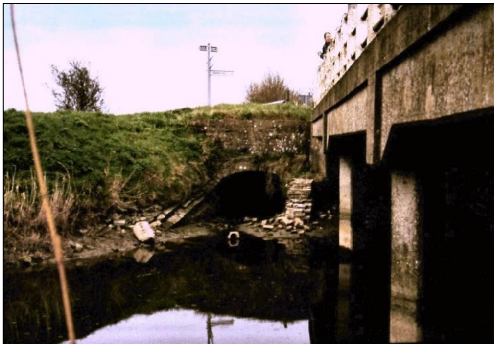
Figure 1: Leeds Gate Bridge and culvert.
