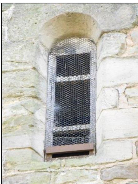
Figures 4 and 5: Modifications were carried out by folding back mesh and removing any sharp edges in various churches to allow bats access into areas where they would not cause the congregation any issues, particularly in the bell tower. These modifications allow access for bats but not problematic bird species such as jackdaws and pigeons.
