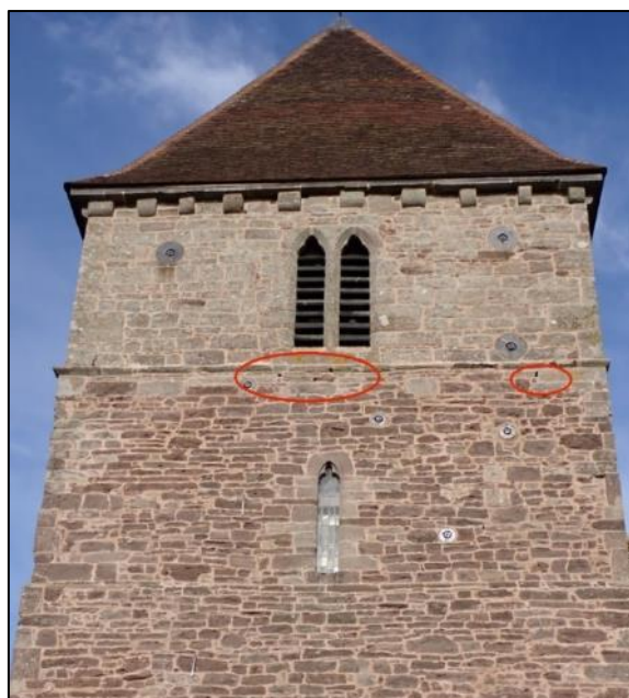
Figure 13: The circled gaps in the masonry were retained during repointing works in 2021, saving existing swift nest sites. Nest sites between the corbels under the eaves were also retained.
