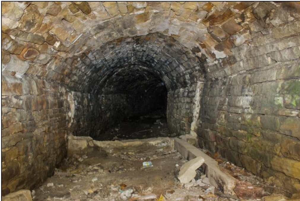
Figure 1: The interior of Rockley Tramway Tunnel.
