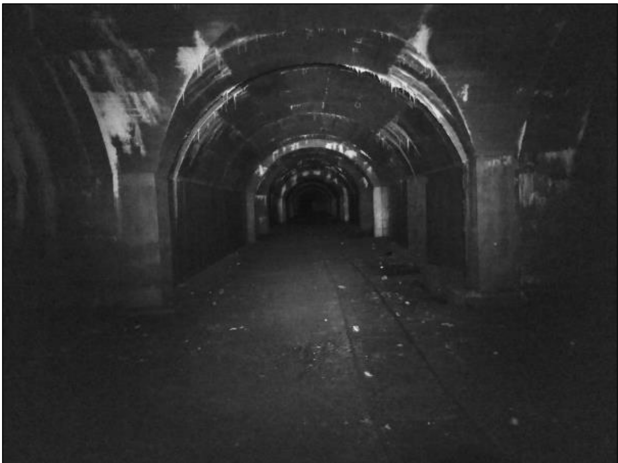
Figure 1: WWII tunnel in Jersey. © Annika Binet.
