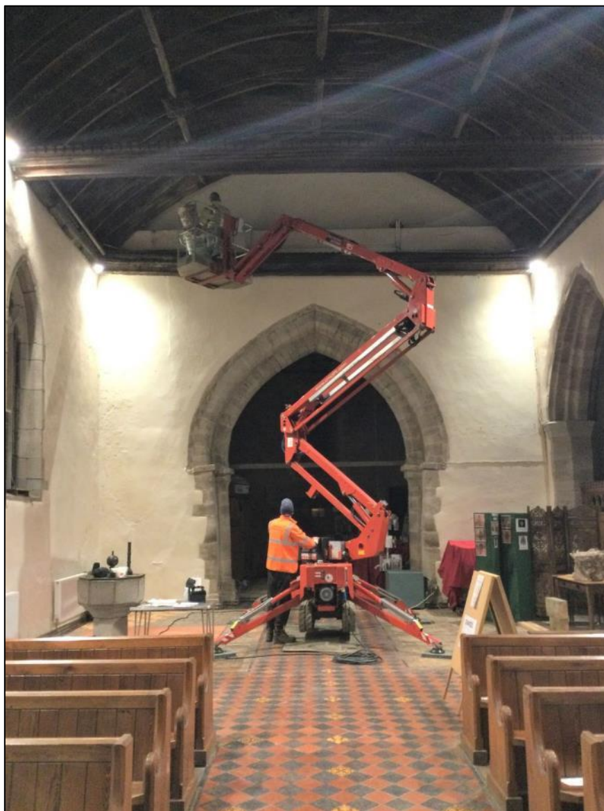
Figure 4: A cherry picker was needed for the works to close bat access to the interior of St Margaret of Antioch.
