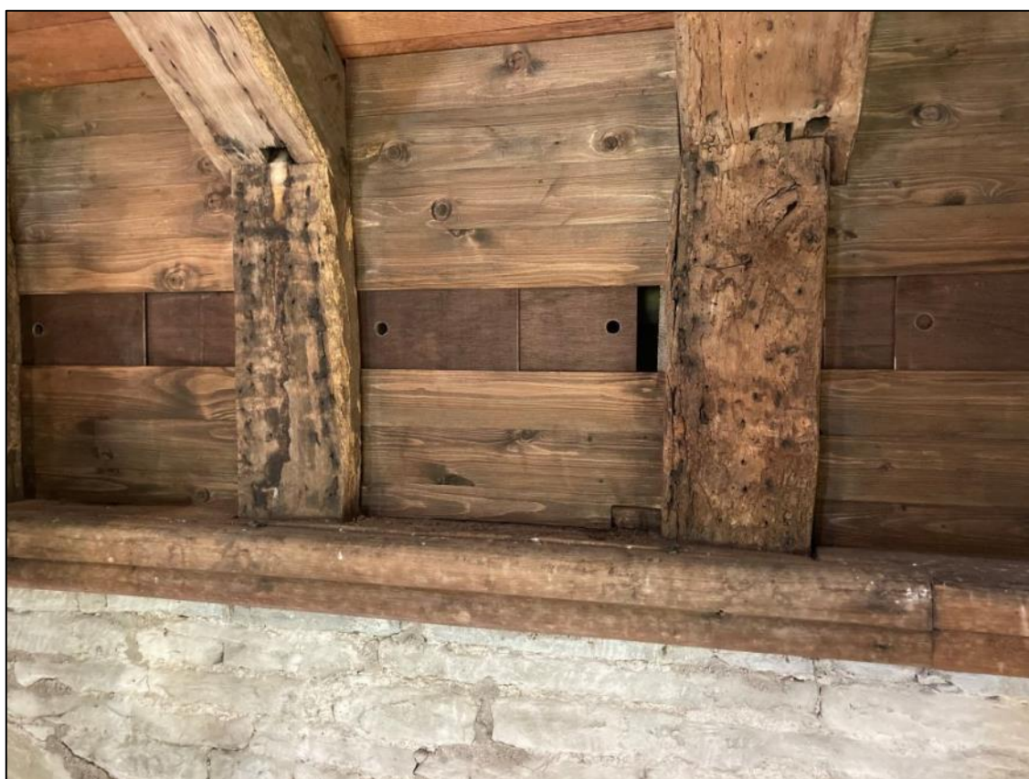
Figure 6: New roost compartments installed at St Mary the Virgin, Pembridge, Herefordshire.
