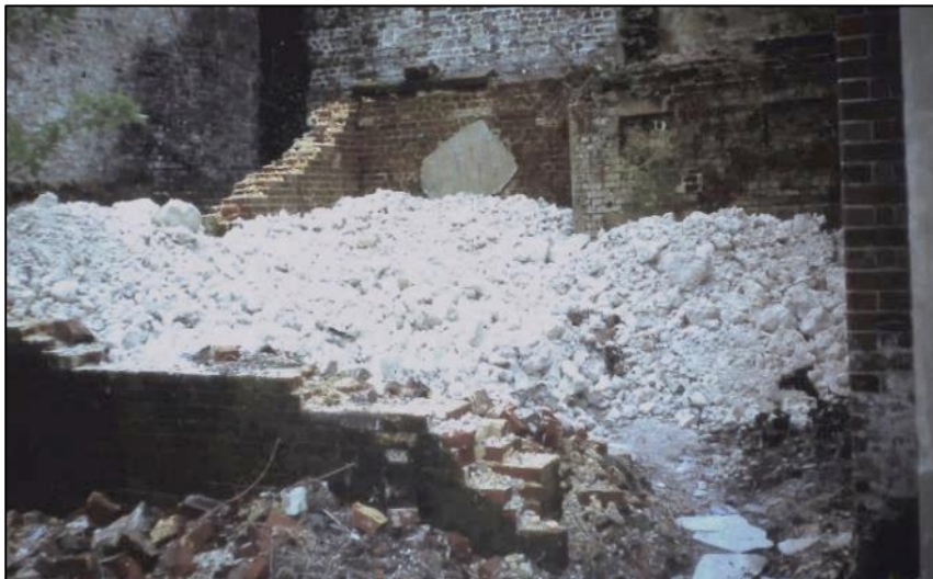
Figure 25: ...and after, approximately 40 tonnes of chalk.
