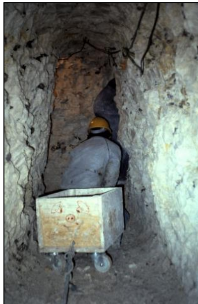
Figure 23. The box on wheels, affectionately known as 'the pig', used to pull out the rubble.
