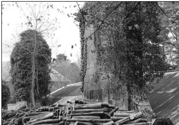
Figure 15: The west elevation roof in the 1970s. Corrugated sheets replaced the slates. In the distance you can make out the roof is 'hipped'. This was changed to a gable during the re-roofing.
