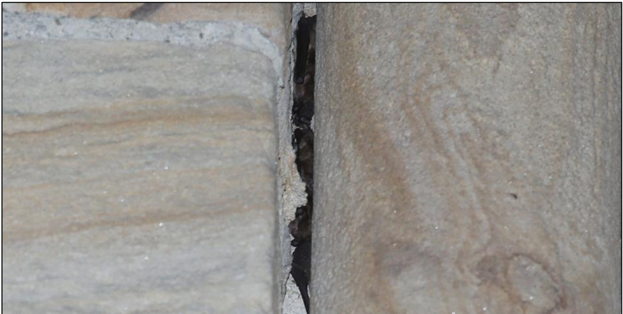
Figure 6: Five bats tucked behind a stone pillar, 12m up. © Neil Tomas.
