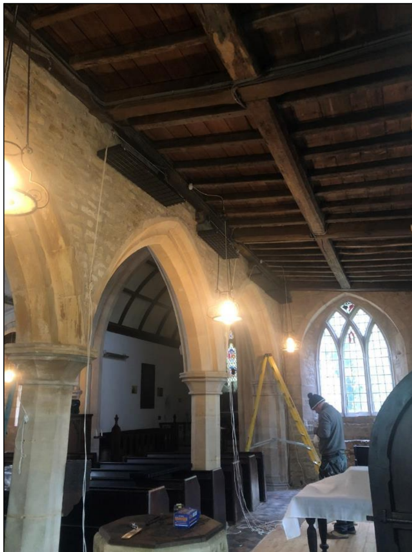
Figure 8: Trays being installed in St Andrew's church, Coston, Leicestershire.
