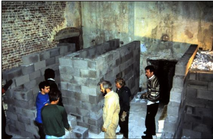
Figure 26: Cave extension (internal) using concrete blocks and polystyrene.
