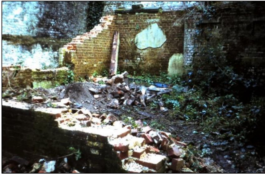
Figure 24: Excavated spoil, before...
