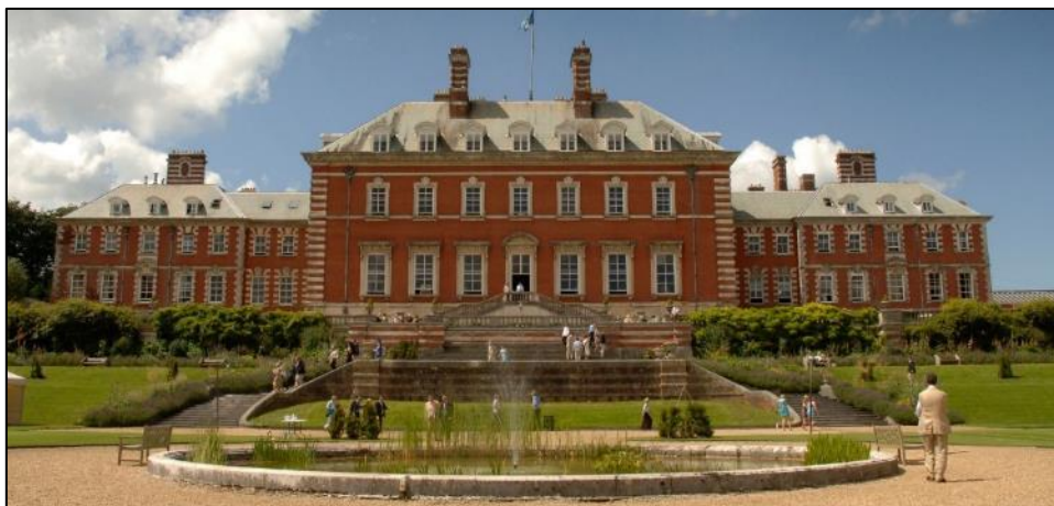
Figure 3: The new house, designed by Norman Shaw, built in a French Renaissance style.
