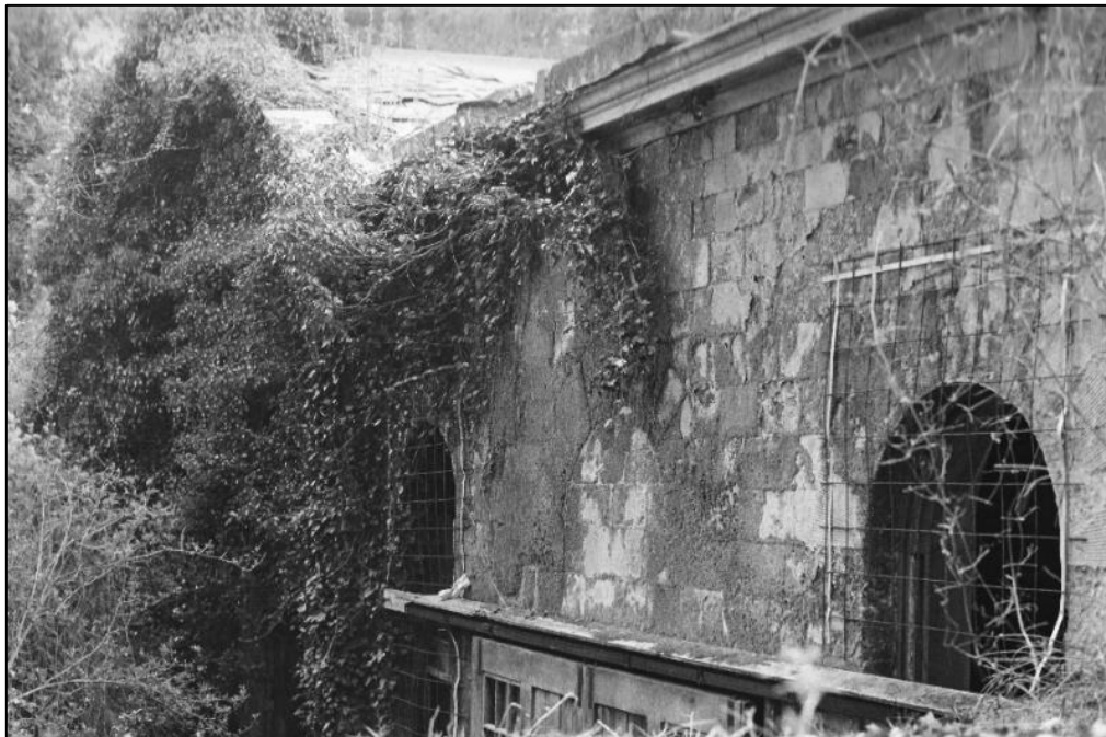
Figure 17: The east elevation in the 1970s. The portico was removed to make rebuilding the roof easier (and cheaper).
