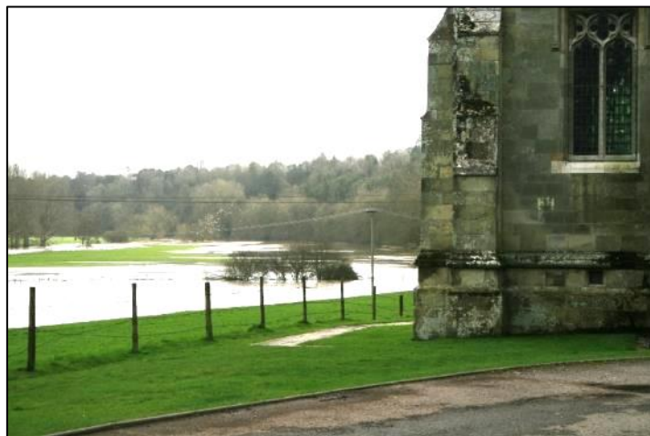
Figure 2: The floods of 2006, showing how close it could come to the house; even after the river had been diverted.
