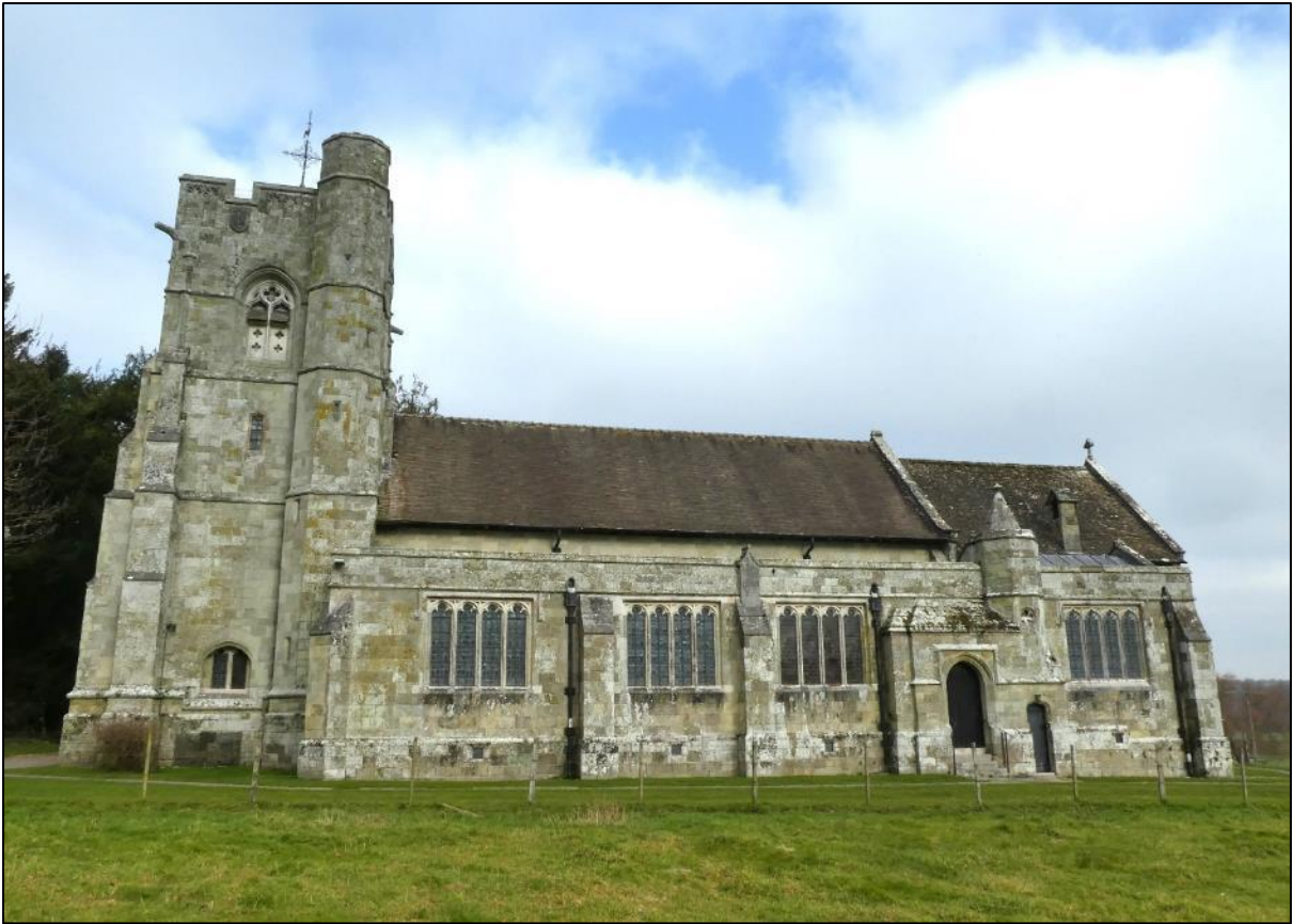
Figure 6: St Martins Church, built from recycled stone, except for the upper, and lower parts of the window frames.
