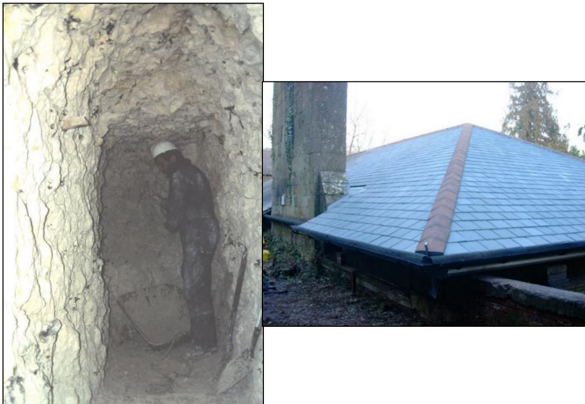
Figure 27: (left) a second, much bigger tunnel was excavated in 1999, by a team of former tin miners from Cornwall, and (right) the final section of roof, on the south elevation.
