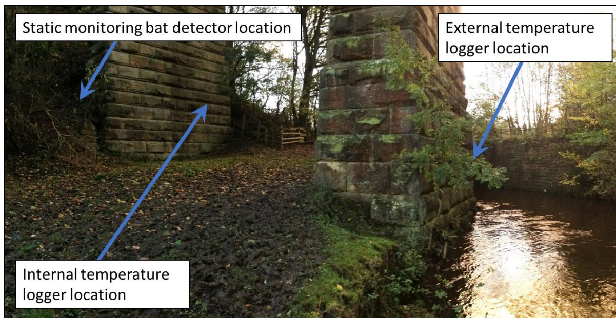
Figure 4: Image showing survey equipment locations.
