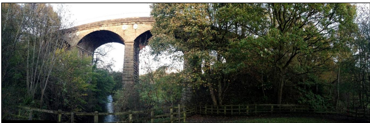
Figure 1: Romptickle Viaduct viewed from the south.
