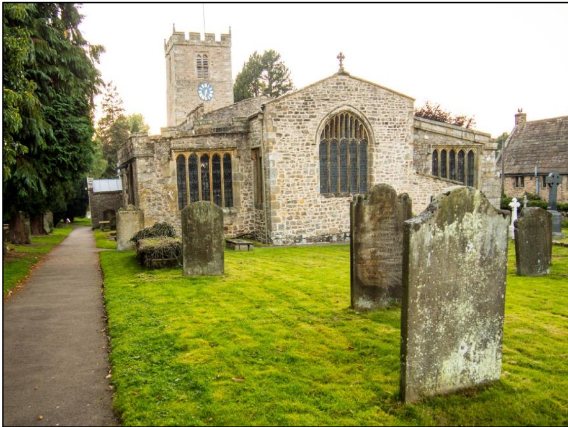
Figure 1: St Andrew's Church Grinton.
