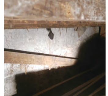
...and low. Lesser horseshoe bats roosting within sections of the original cellar.
